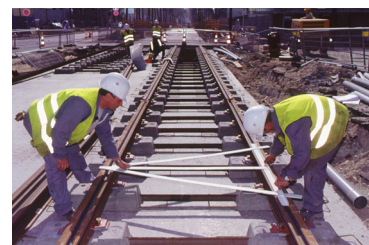
Chantier TRAM, Mulhouse Source : SITRAM
