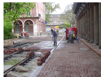
Chantier TRAM, Mulhouse Source : SITRAM
